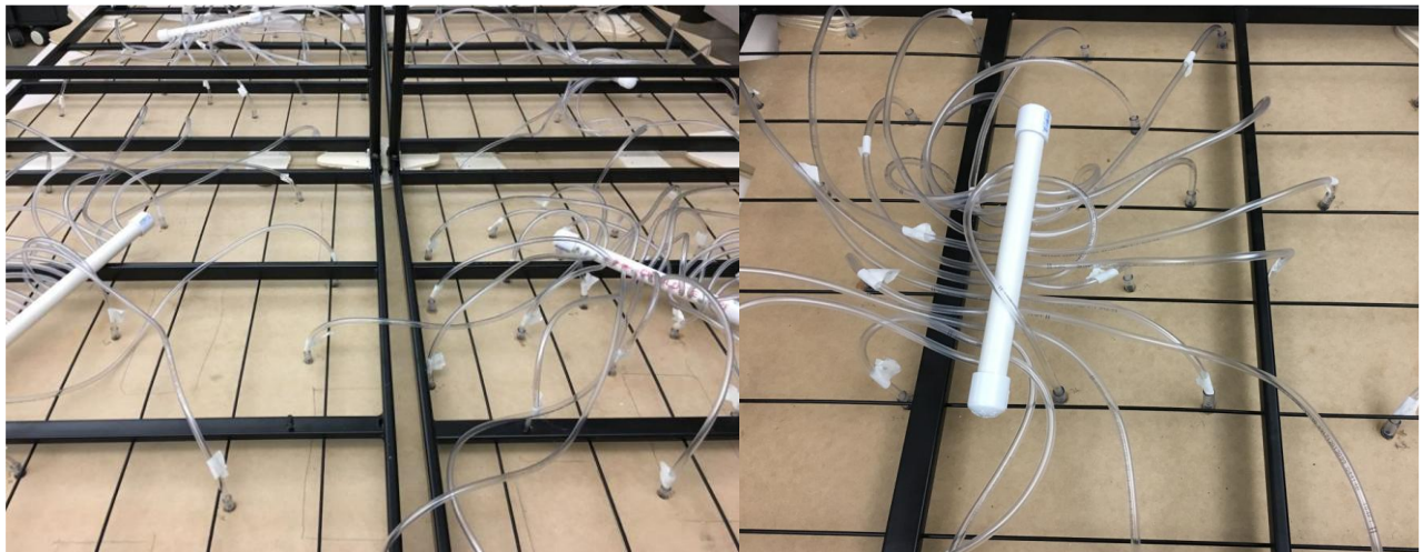
[Figure 78] The tubing under the floor. Each manifold is working for a separate zone and for a single solenoid valve that would be controlled separately. (Author, 2017)
